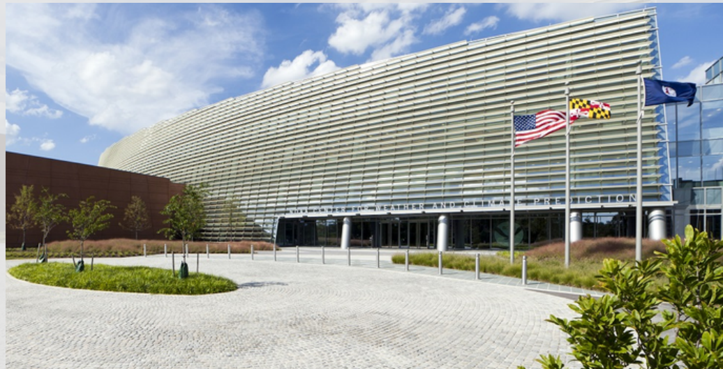
Front view of the NOAA Center for Weather and Climate Prediction (NCWCP) building in College Park, Maryland.
